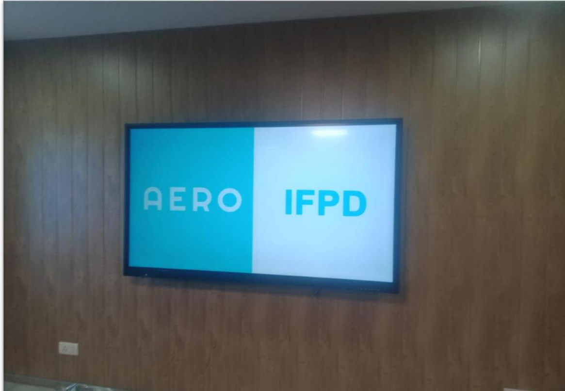
75" Inches Interactive Display Installed at Furniture Store, Kirti Nagar - Delhi
