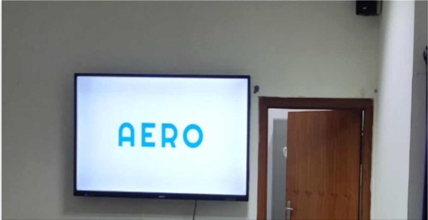
75" Inches Interactive Display Installed at Bird Research Center CRAI, Bareilly
