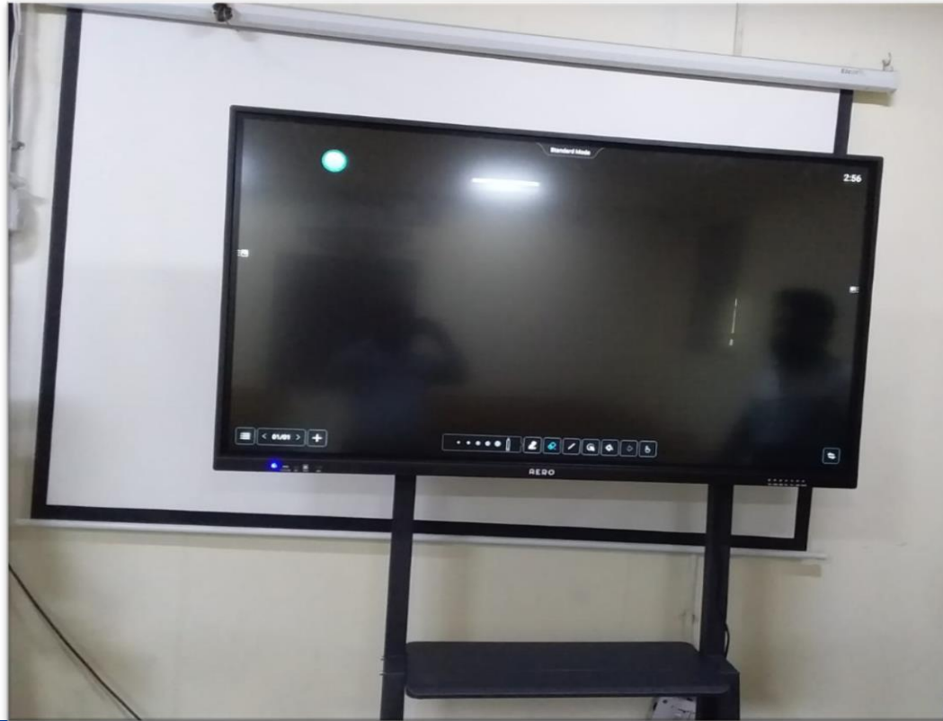
2 NO.S 65" Inches Interactive Display Installed at Homeopathic Hospital, Delhi
