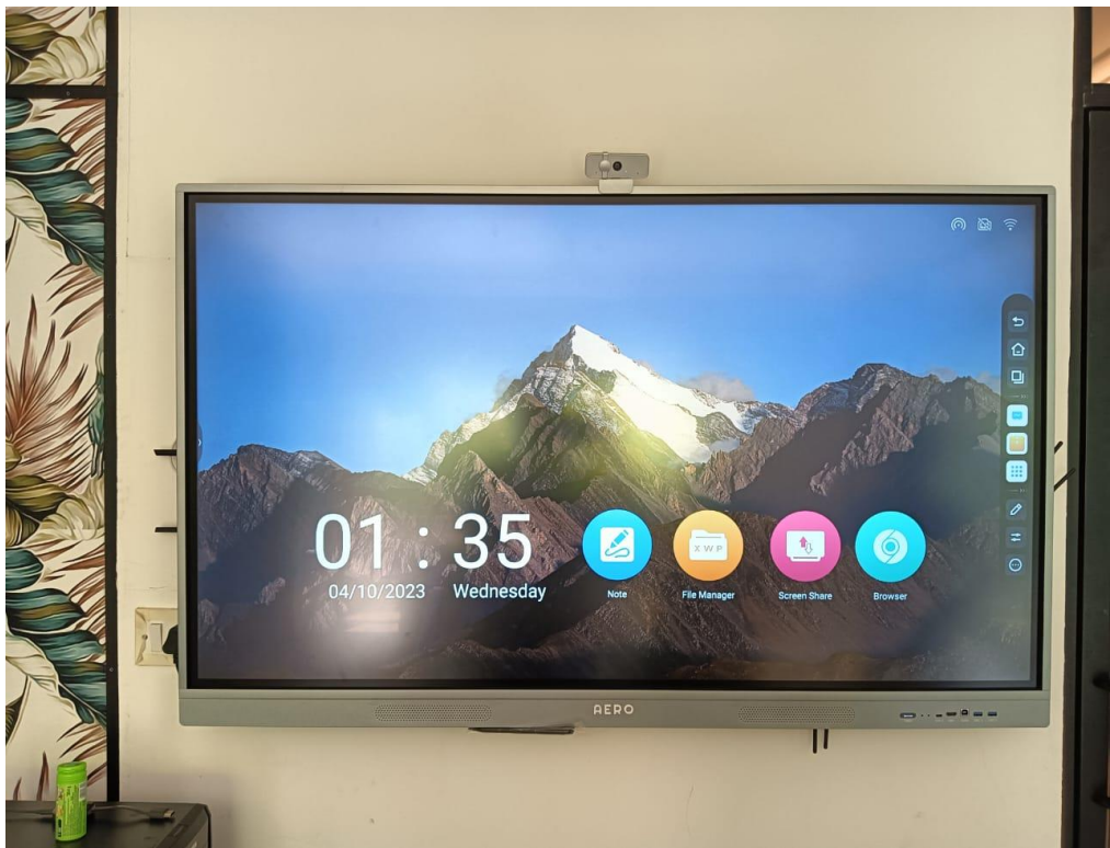
3 NO.S 75" Inches Interactive Display Installed at Base Hospital, Delhi Cantt - Delhi
